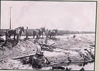
Repairing the dike after the hurricane of 1926.
