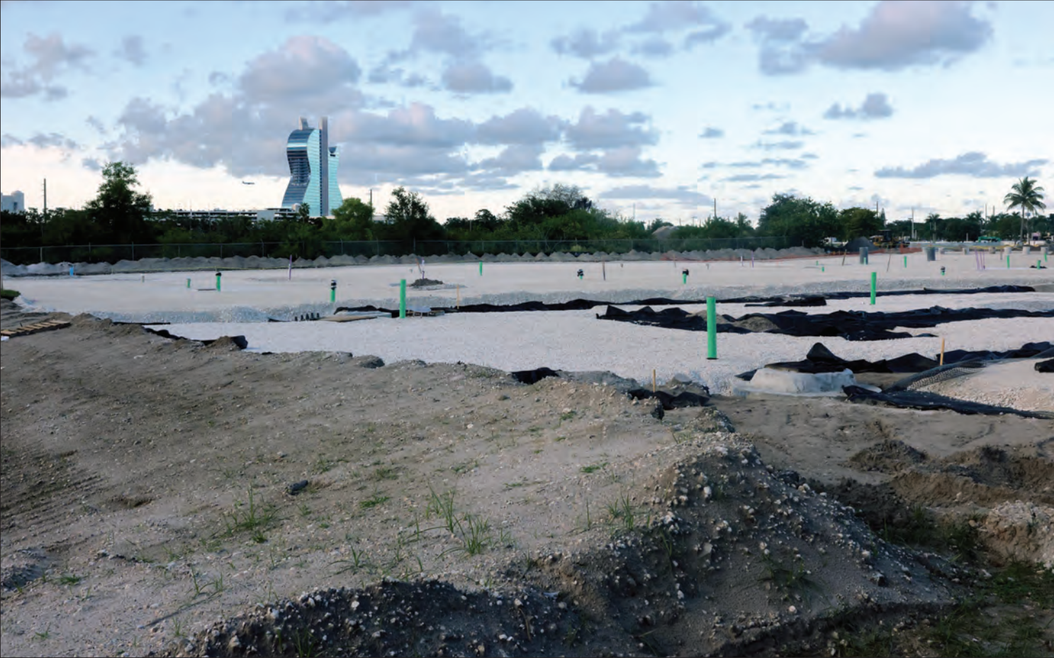
Above and below, the Community Center.
