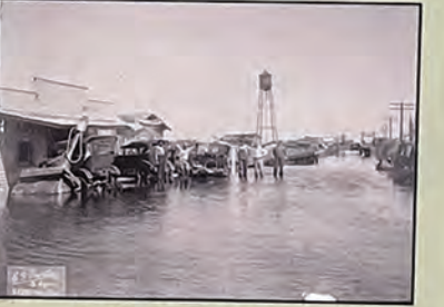
Flooding after the 1926 hurricane.
