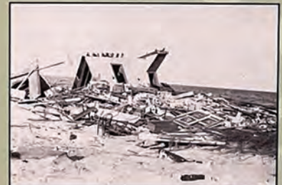
Damage after the 1928 Okeechobee Hurricane.
