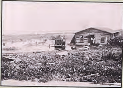
Breaks in the low earthen dike caused flooding throughout the area.
